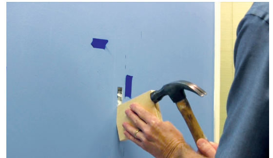
Step 2: Start rough opening with wood scrap
