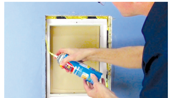
Step 9: Seal interior with low-expansion foam
