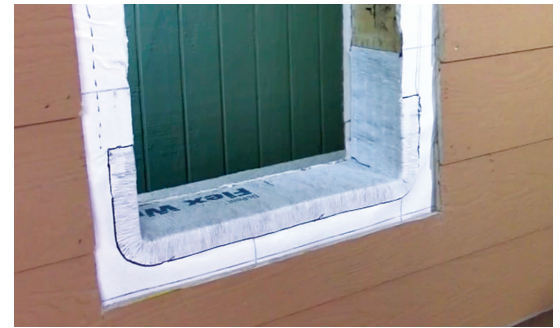
Step 7: Properly prepare rough opening
