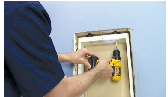
Step 8: Attach door through head jamb
