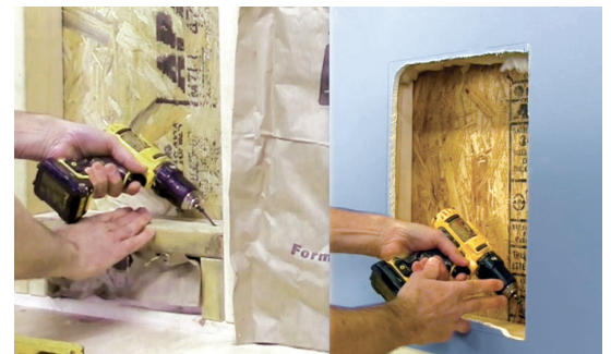
Step 4: Install risers and sill
