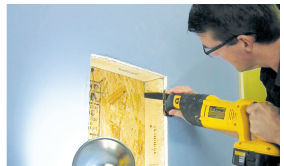
Step 5: Cut exterior opening
